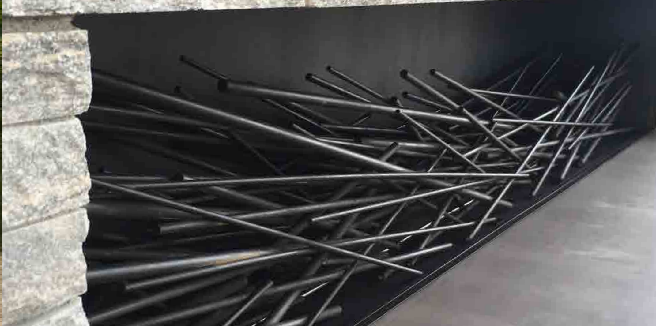
BLACKENED MILD STEEL CROSS-HATCH BRANCH INSERT
