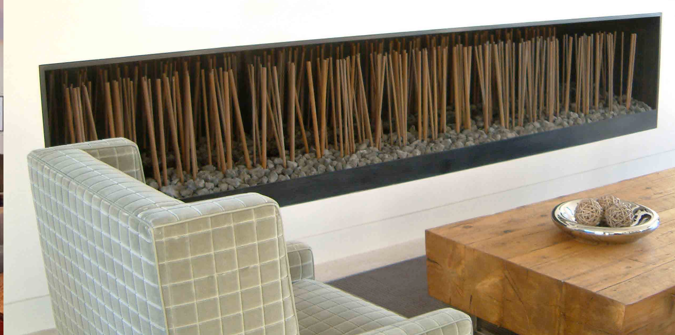
66 BLACKENED STEEL FIREBOX w RUSTED STEEL GRASS INSERT
